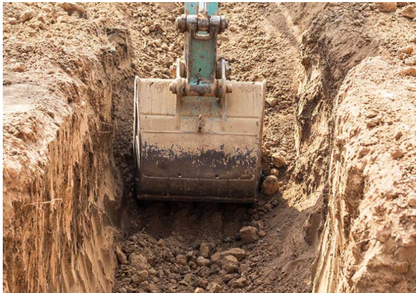
Plate 4.3: Traditional excavator bucket (Downer, 2022)
