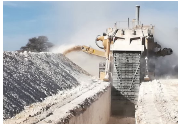
Plate 4.4: Chainsaw trencher (Downer, 2022)
