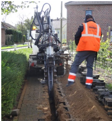
Plate 3-2: Integrated Trenching Wheel
