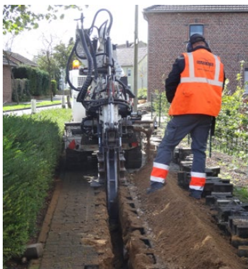
Plate 2.4: Integrated Trenching Wheel
