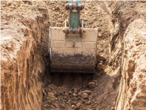
Plate 2.5: Traditional Excavator Bucket (Downer, 2022)
