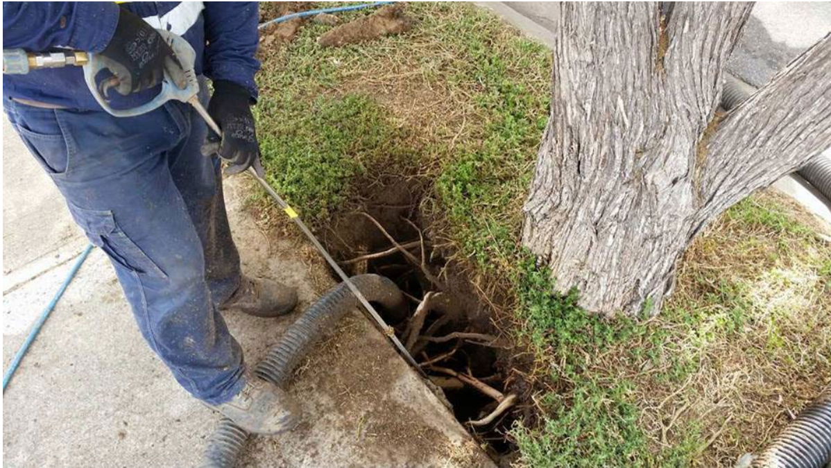
Plate 2.8: Water Excavation to Investigate Tree Root Depth and Extent (South Vac, 2023)
