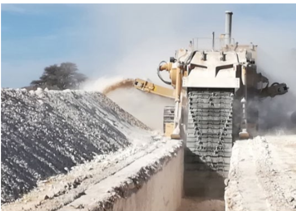
Plate 2.6: Chainsaw Trencher (Downer, 2022)
