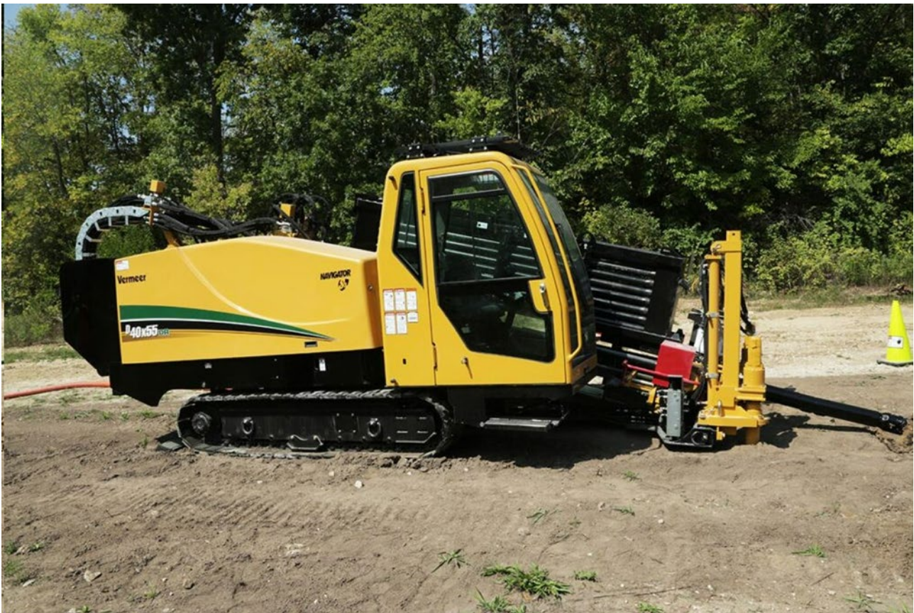
Plate 2.7: HDD Installation (reference)
