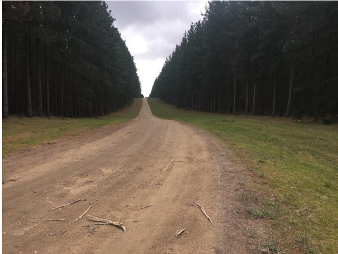
Dewars Road, facing north (Source: AECOM photo taken 30/07/2020)
