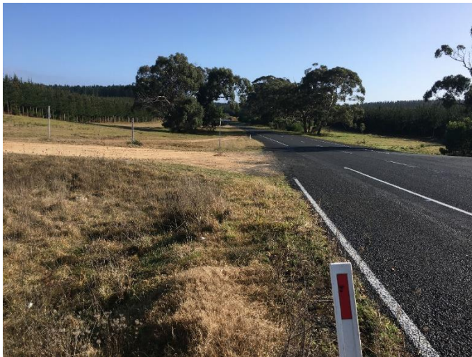
Wilsons Lower Road intersection, facing north (Source: AECOM photo taken 30/07/2020)
