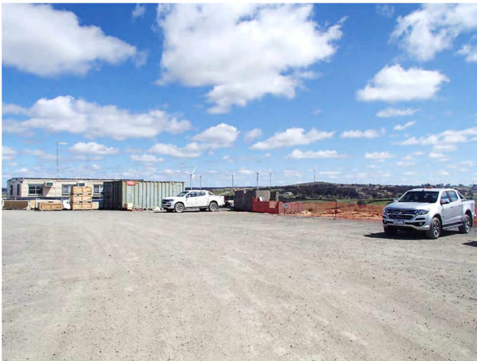
Plate 14 Typical contractors site office and amenities compound (Image: ©GBD 2023)
