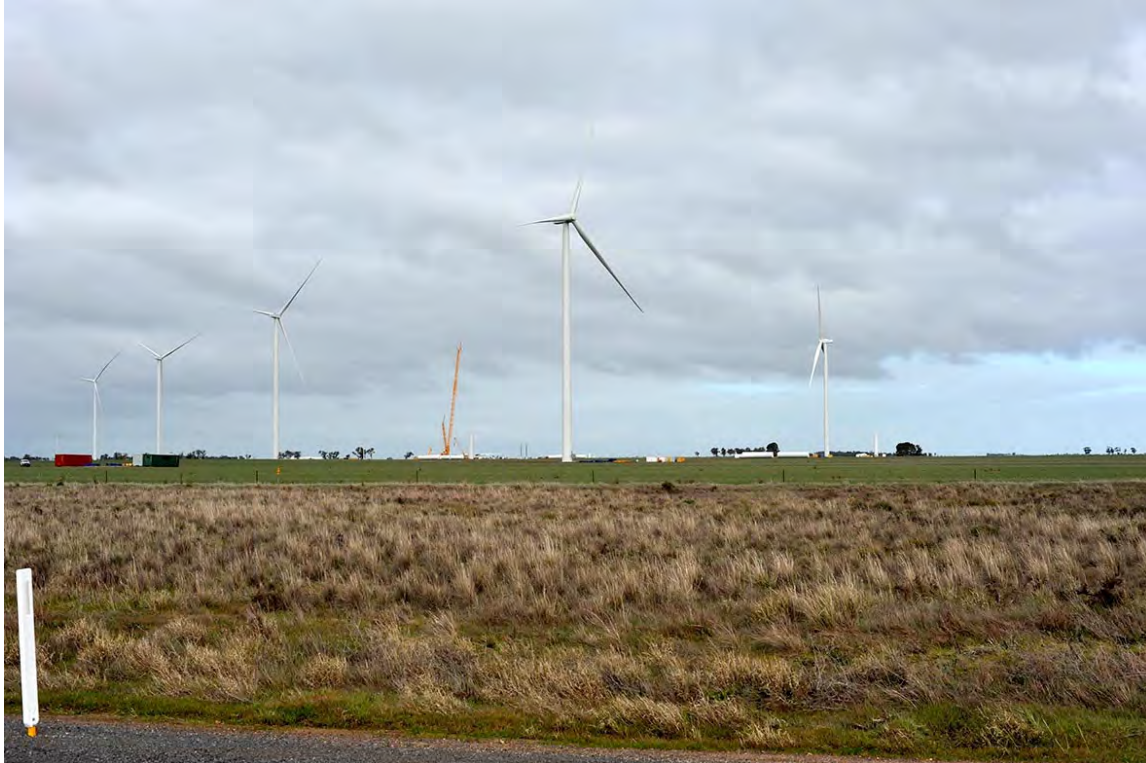
Plate 9 – Murra Warra wind farm under construction (Image: ©GBD 2017)
