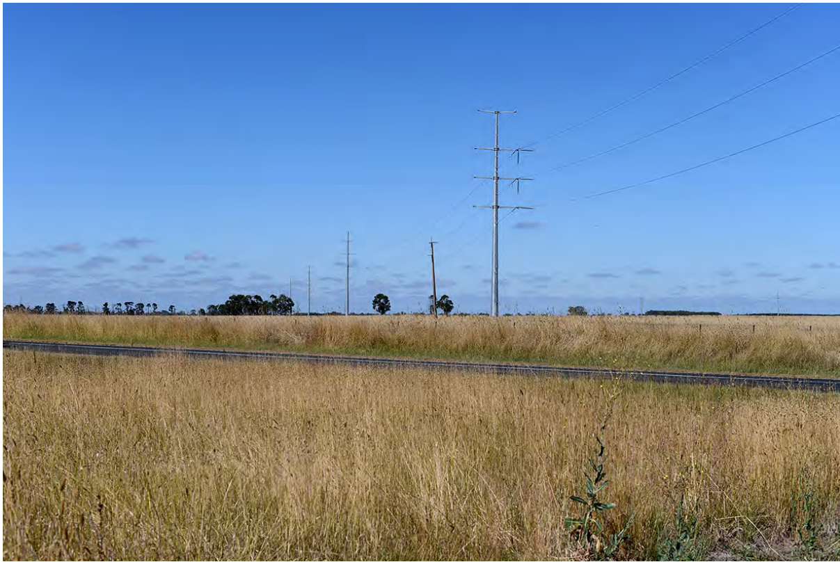
Plate 6 – View toward existing wind farm transmission line infrastructure, Mortlake (Image: ©GBD 2023)
