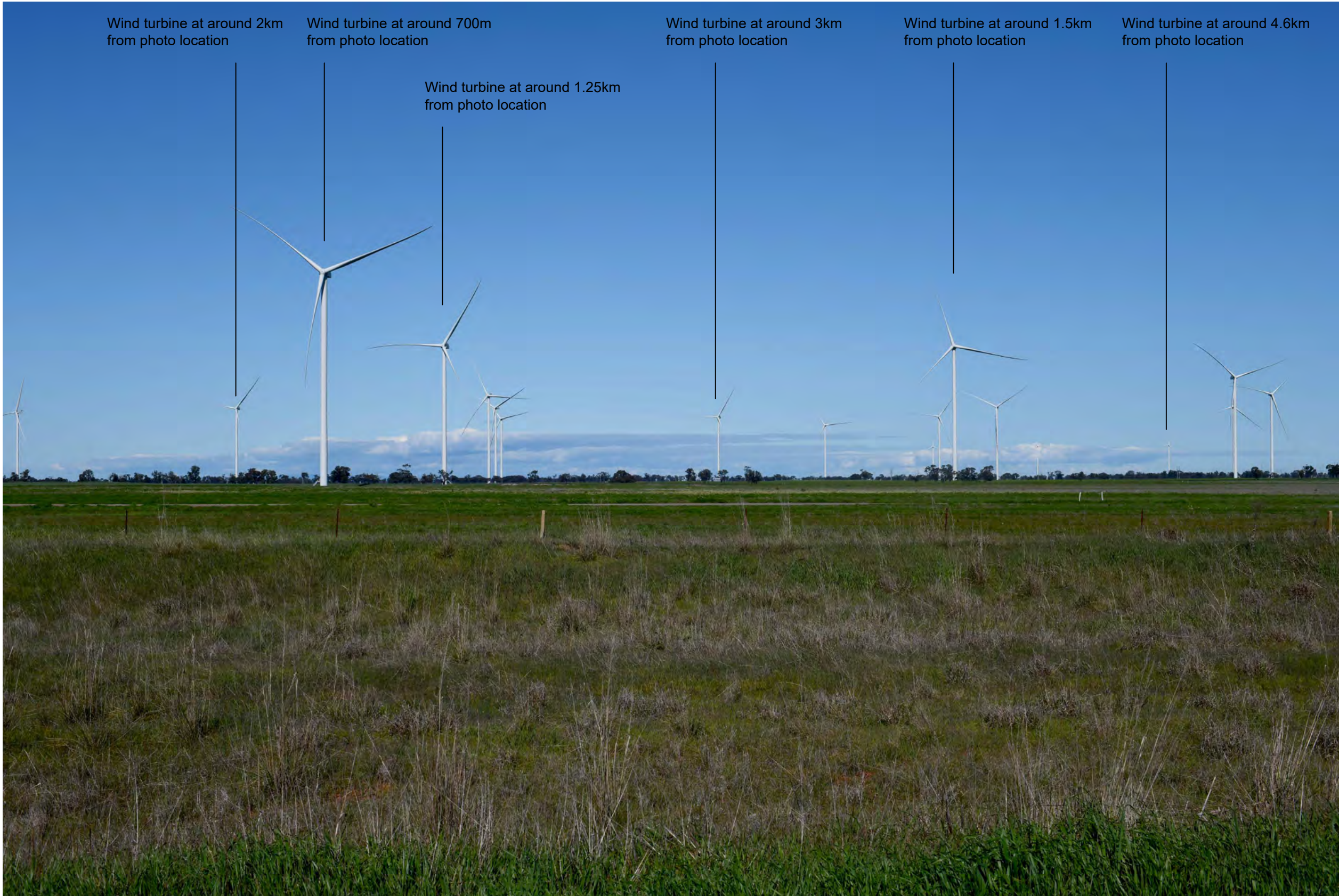
View south from Barrat Road toward Murra Warra wind turbines GDA94, Zone 54, E: 621714 N: 5971935 Camera Nikon D850, 50mm focal length Date 9 August 2022, Time 12:10pm Murra Warra wind turbine: rotor diameter 144m, hub height 139m and tip height 211m
