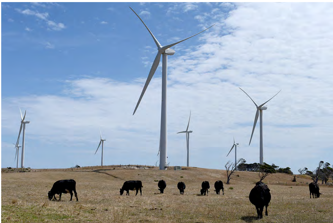
Plate 2 – Typical wind turbine structure (REpower MM82 with 69m hub height and 82m rotor diameter) and hardstand, Cape Bridgewater (Image: ©GBD 2023)
