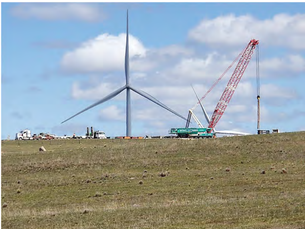
Plate 12 Typical crane plant utilised in wind turbine construction (Image: ©GBD 2023)
