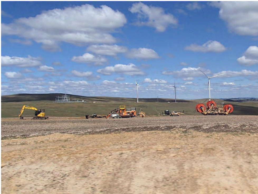
Plate 11 Cable laying equipment (Image: ©GBD 2023)
