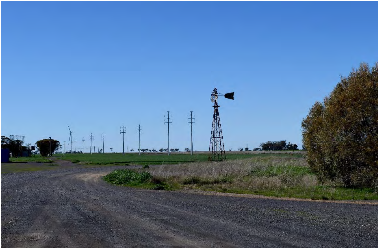
Plate 5 – View toward a double 220kV transmission line at Murra Warra wind farm (Image: ©GBD 2022)
