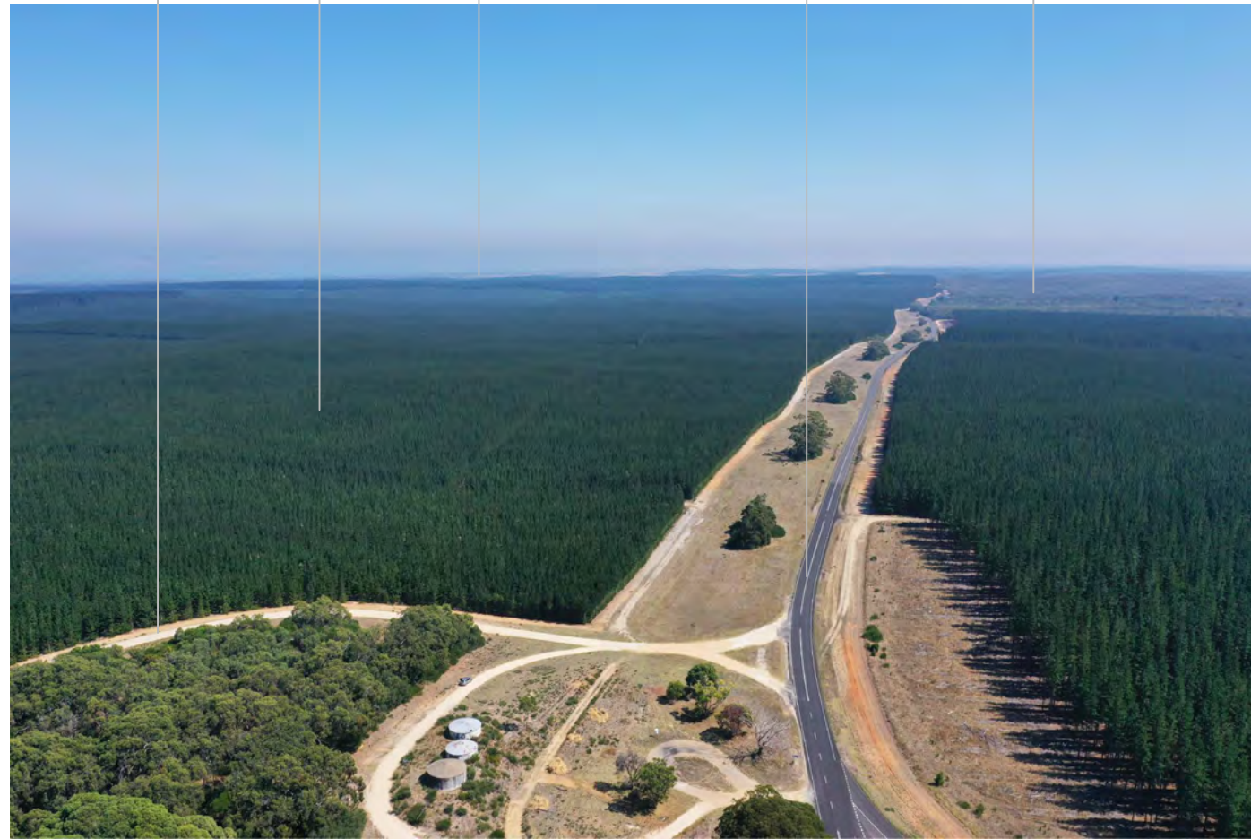
Aerial Photo Location A6- View west from above Portland Nelson Road corridor
