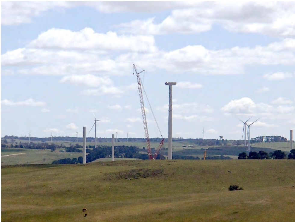
Plate 15 Typical view toward wind turbines under construction (Image: ©GBD 2023)
