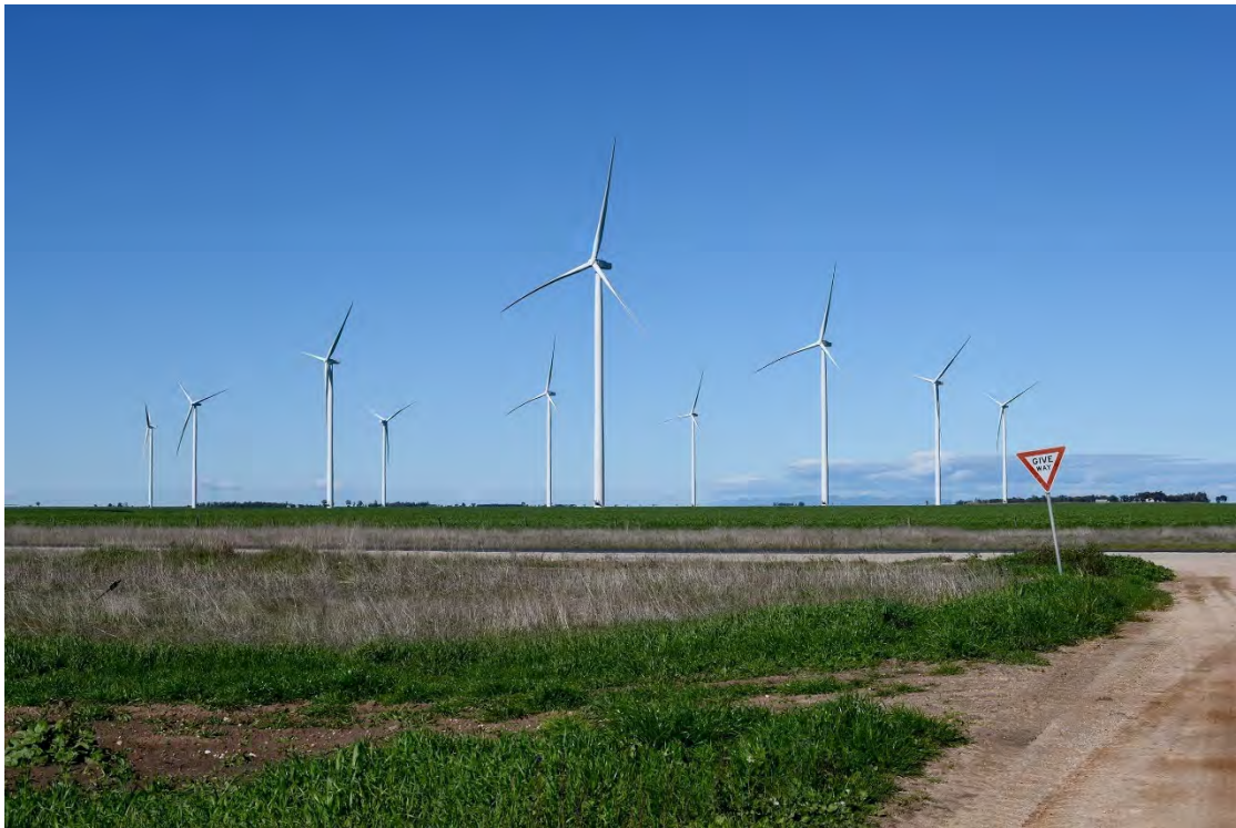
Plate 1 – Typical wind turbine structure (139m hub height and 158 rotor diameter) Murra Warra Wind Farm, Murra Warra VIC (Image: ©GBD 2022)
