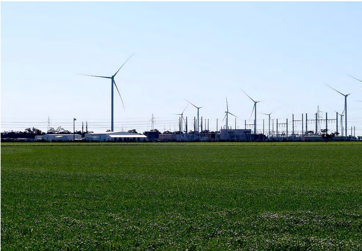
Plate 8 – Main substation and operations centre, Murra Warra Wind Farm, Murra Warra VIC (Image: ©GBD 2022)
