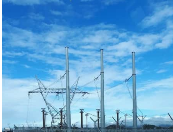
Figure 4 – Typical UG/OH Transition Station (with example photos)
