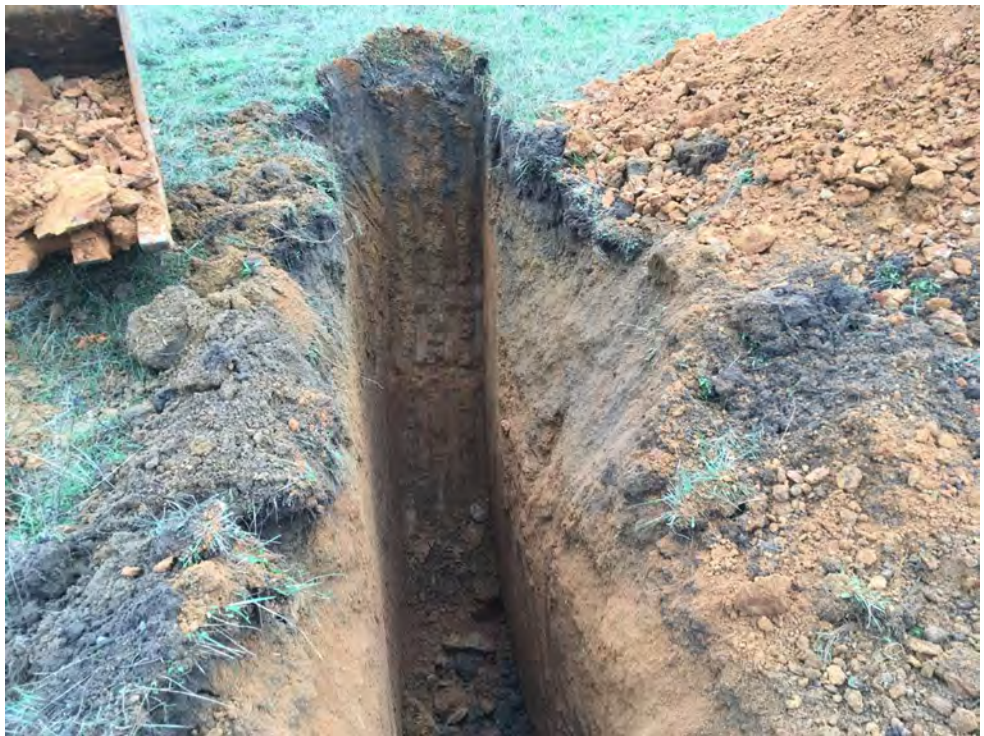
Photo: 14 Date: 13/05/2021 Description: TP16
