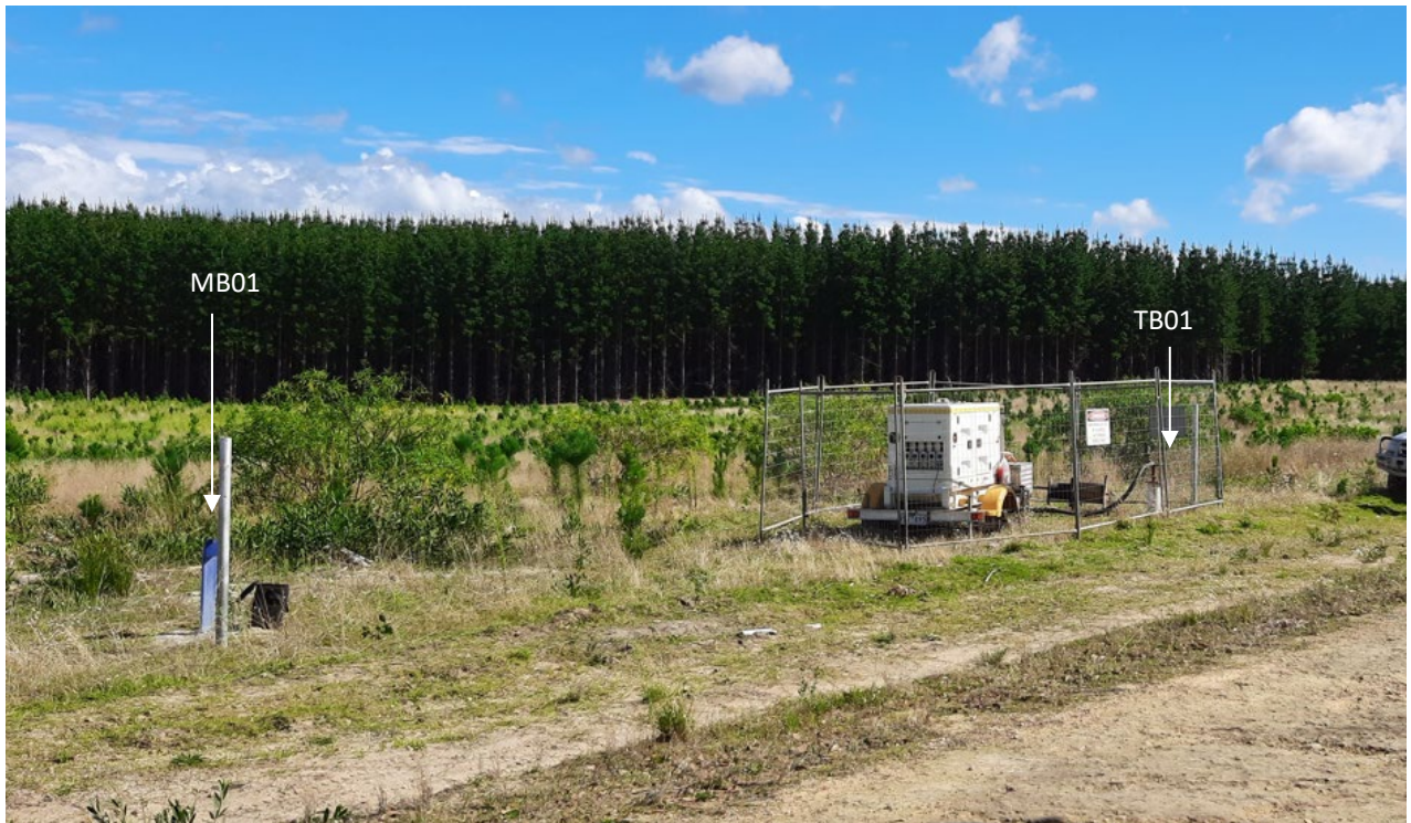
Plate 1 Site layout showing TB01 and MB01 with pump and generator
