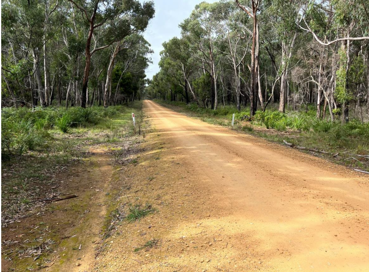
Figure 8 One of the many minor drainage lines that cross Boiler Swamp Road and is considered suitable for open cut, trenched crossing construction methodology (white culvert markers).
