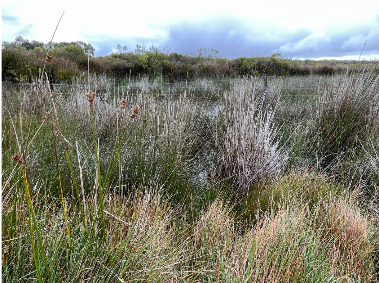
Figure 6 Visible ponding of the north side of the farm access track and project boundary.
