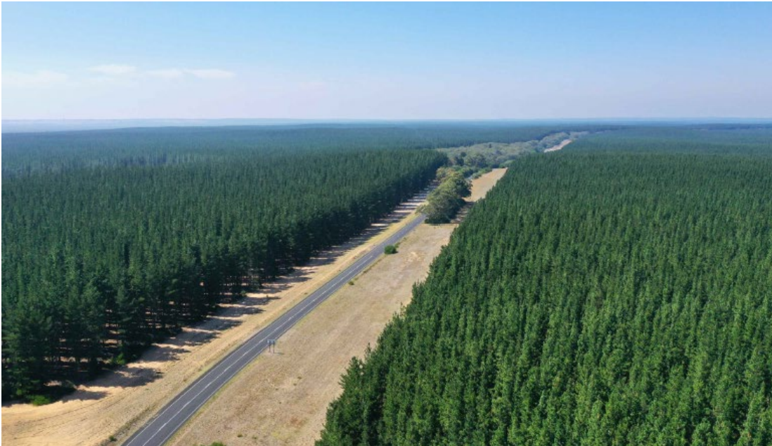
Figure 2 Aerial photo of the pine plantation in the Kentbruck area, which represents common landscape features surrounding the Project Area. Portland-Nelson Road is also shown in this photo
